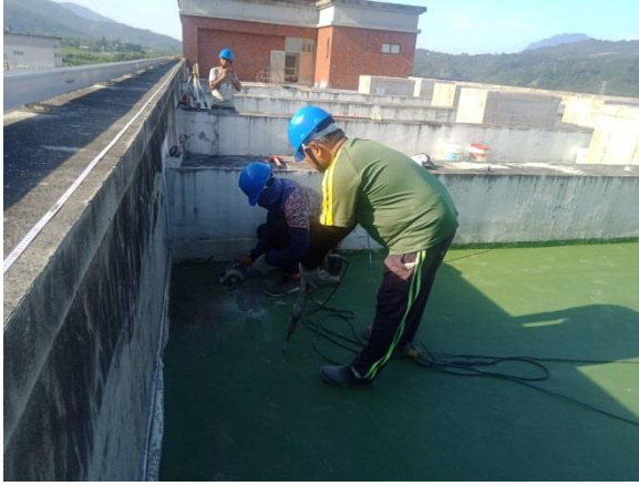
Administrative building roof waterproofing work
